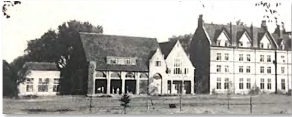
South Elevation of Geography Room in 1937 positioned at right angles to the west end of the Ibberson Building
